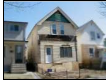
HOP home before renovations
