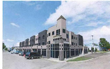
Affordable Housing Gaetz Landing Phase 2
