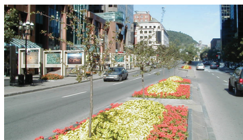
High quality streetscape design (Median, sidewalks and street furniture)
