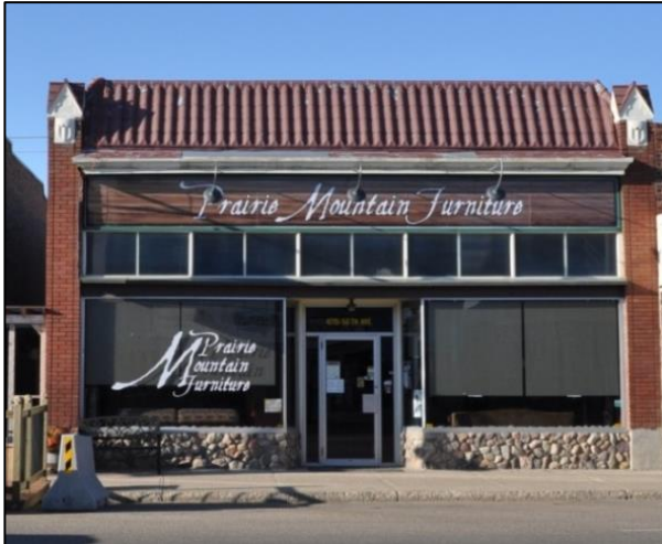
View from the north of existing building (RKH Architecture, June 2012)
