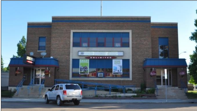
View from the south of existing building (RKH Architecture, June 2012)
