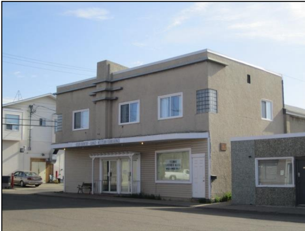
View from the southwest corner of existing building (RKH Architecture, June 2012)
