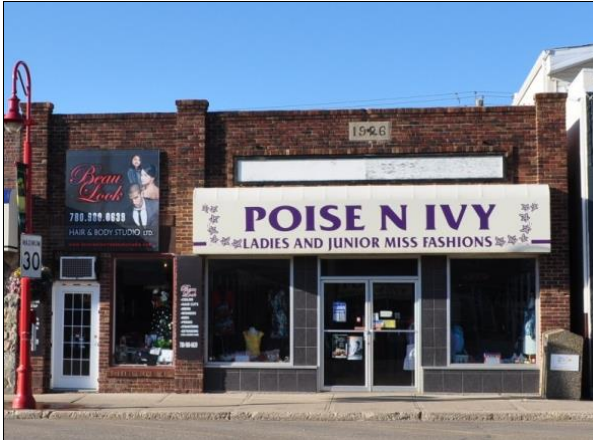
View from the north of existing building (RKH Architecture, June 2012)
