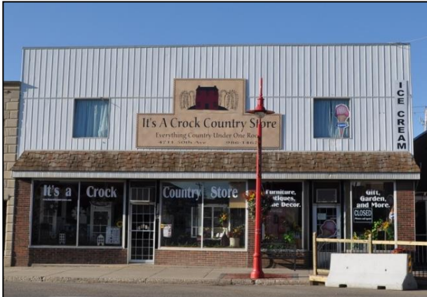
View from the north of existing building (RKH Architecture, June 2012)
