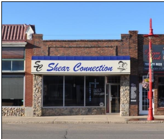
View from the north of existing building (RKH Architecture, June 2012)
