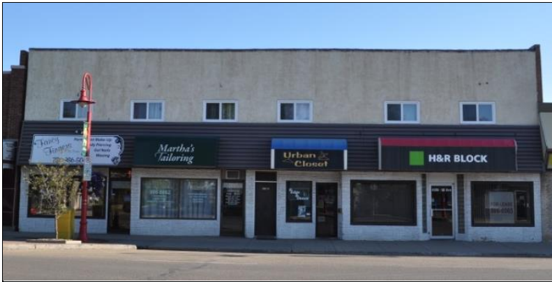
View from the south of existing building (RKH Architecture, June 2012)
