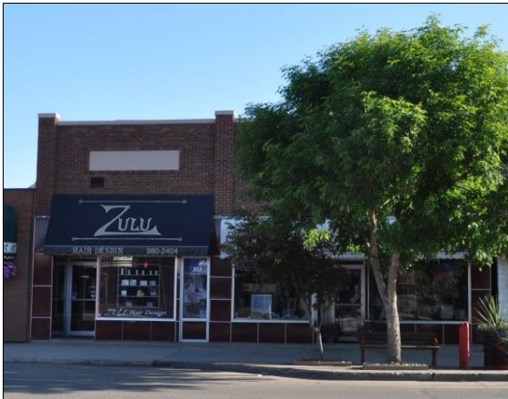
View from the south of existing building (RKH Architecture, June 2012)
