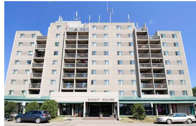
Rooftop telecommunication antennas on Summit Square Apartments, Leduc, AB
