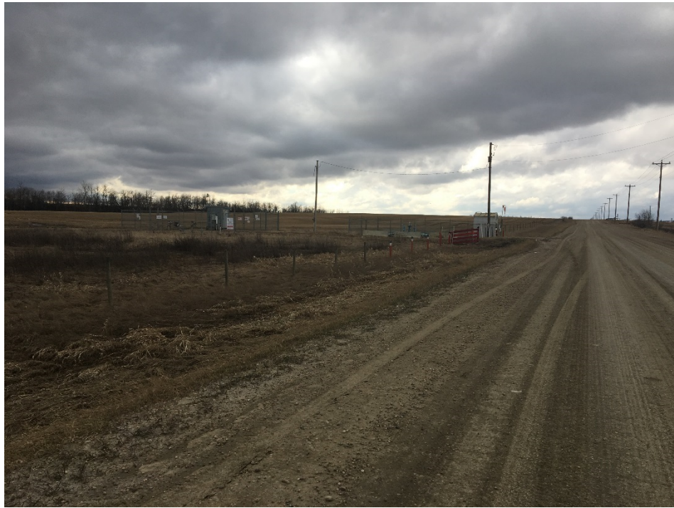
View showing existing valve station
