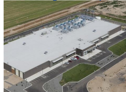
Data Storage & Computer Centres
