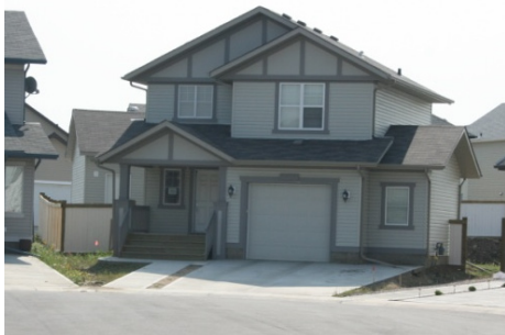
Example of a front-attached garage integrated into the façade of the single-detached home. Edmonton (source: Jennifer Cardiff)
