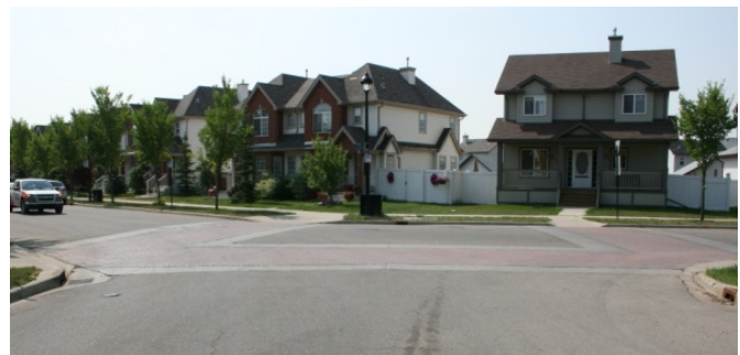
Example of special pavement treatments to designate pedestrian crossings. Edmonton (source: Jennifer Cardiff)
