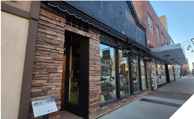
Parapets And Projecting Signage
